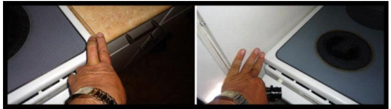
Electric, Improper clearance.
