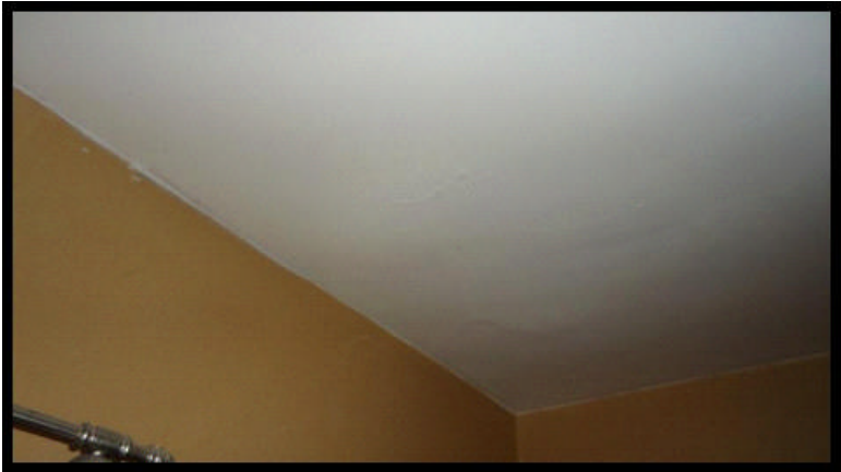
Previous Leak - There are signs of a previous water leak in the ceiling in this room. It does not appear to be an active leak.
