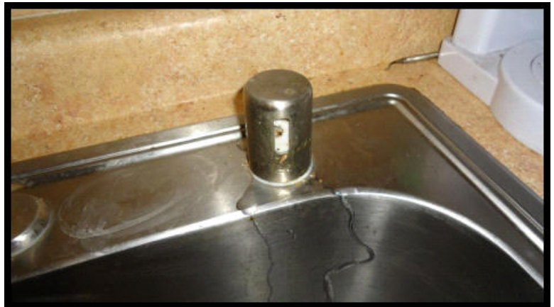
Backing up though air gap.
