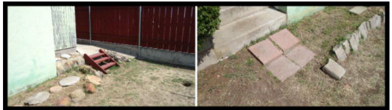
Handrails needed, Improper rise/run on steps.
