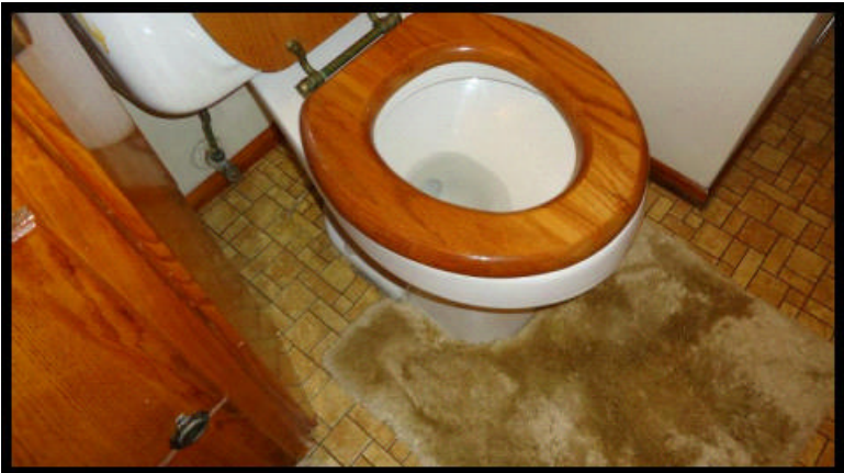
The following problems were noted at the toilet: Toilet is loose at floor.
