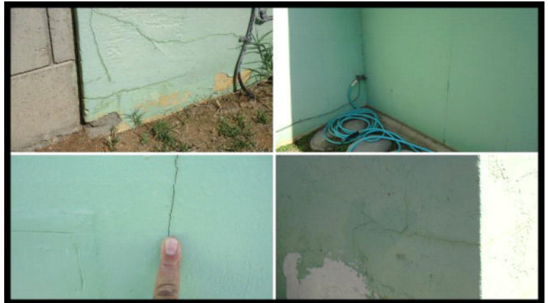
Cracks noted are major, Damaged siding.
