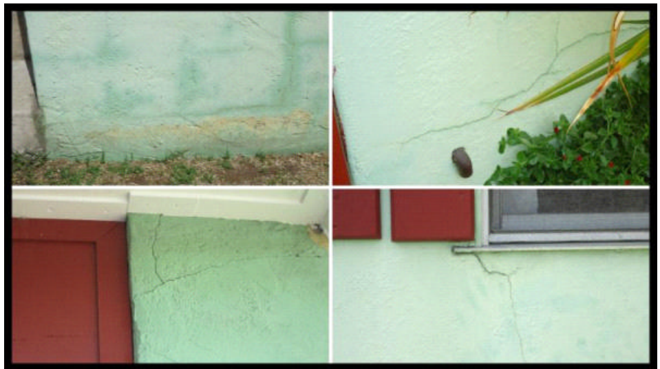
Cracks noted are major, Damaged siding.
