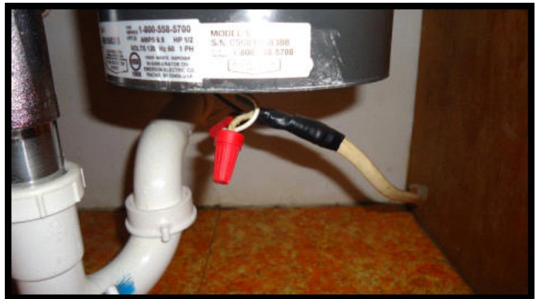
Improper wiring.
