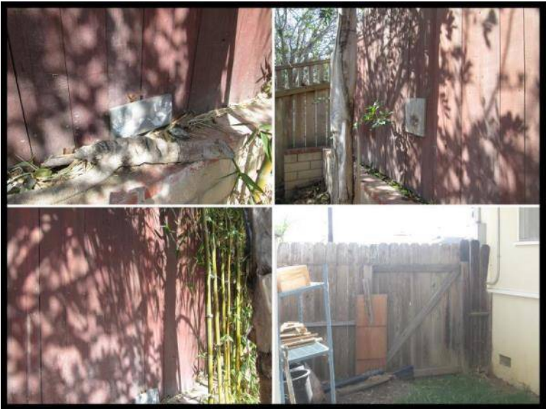
Damaged Gate needs repair or adjustment, Loose/rotted posts.
