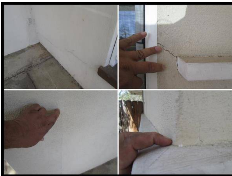
Cracks noted are major, Damaged/rotted from moisture.
