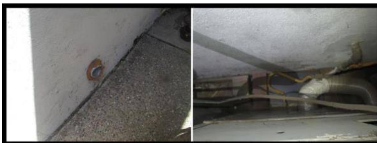
Improper seal, trimmed.
