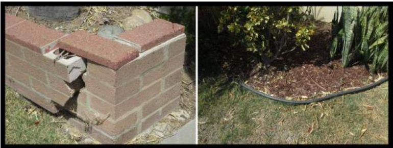
Displacement/Cracks major. Barrier holding moisture next to walls.
